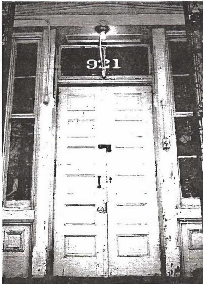
Figure 46 North Wood Entrance Portico and Door Detail.
