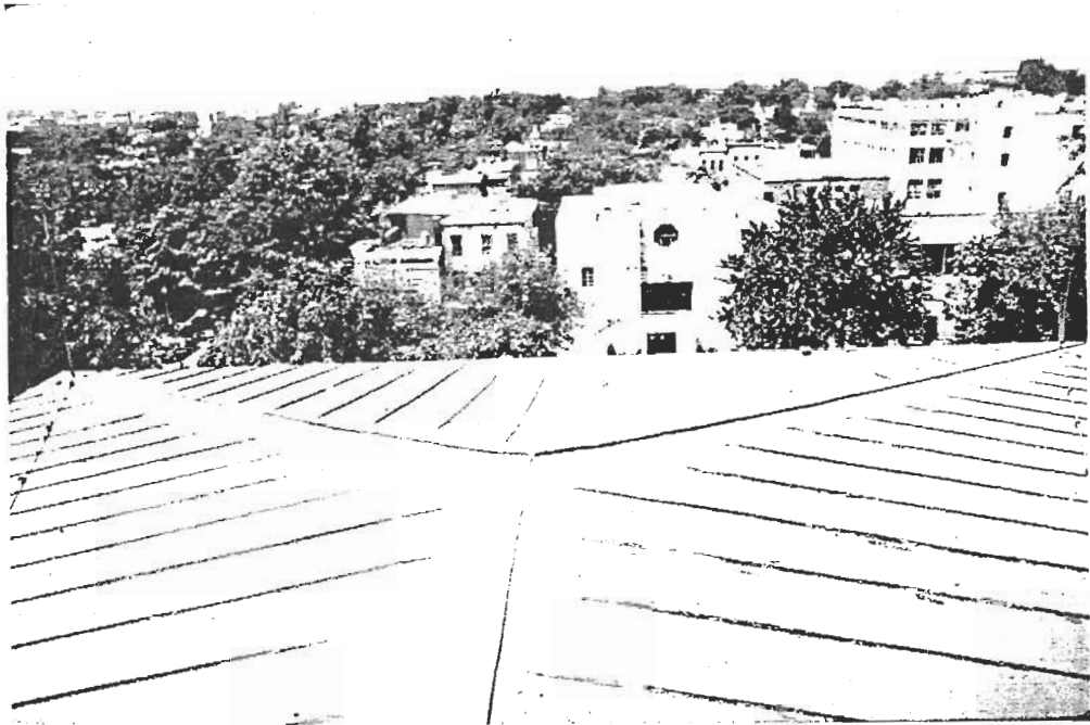
Figure 97 East View of Standing Seam Metal Hipped Roof.
