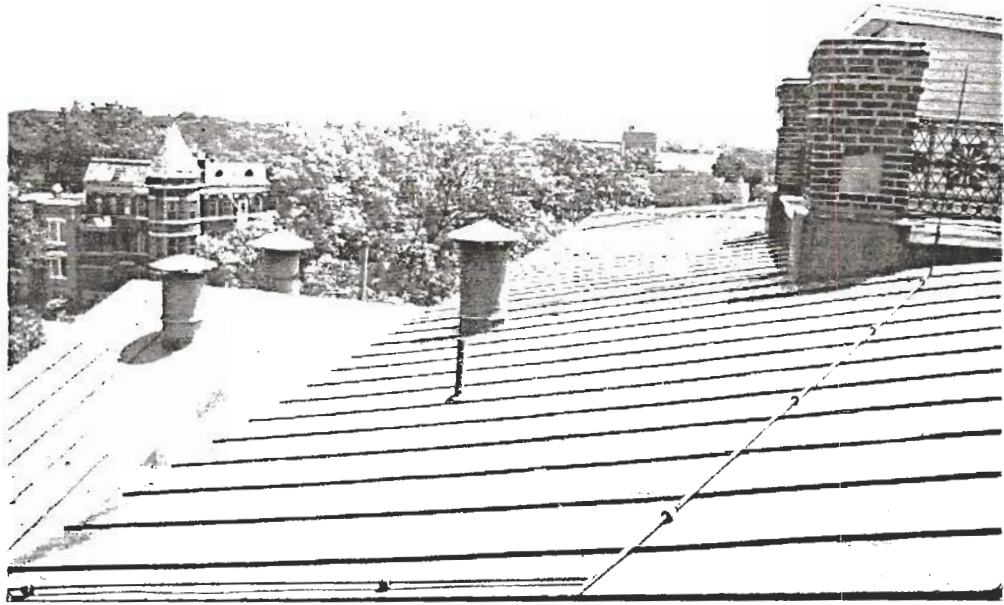
Figure 96 Standing Seam Metal Roof/Chimney Vent Detail Overlooking North Pediment.
