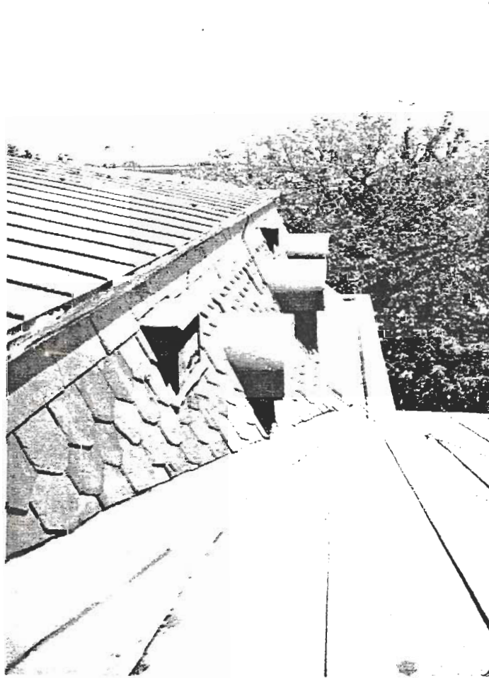
Figure 103 Southeast Elevation at Mansard Roof and Dormers (Note A/C Openings).
