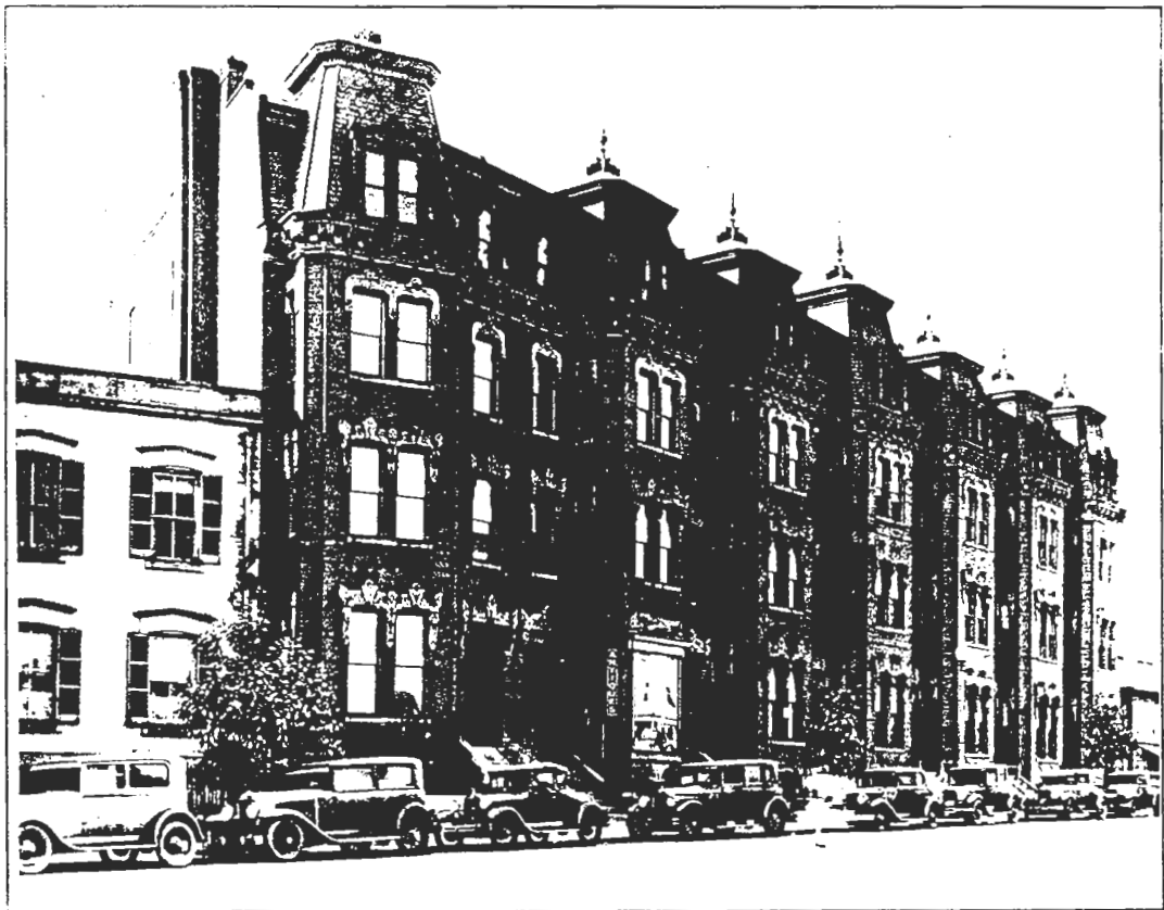
Figure 9 Photograph of Phillips Row (1302-1314 Connecticut Avenue), 1929. Goode, Capital Losses.
