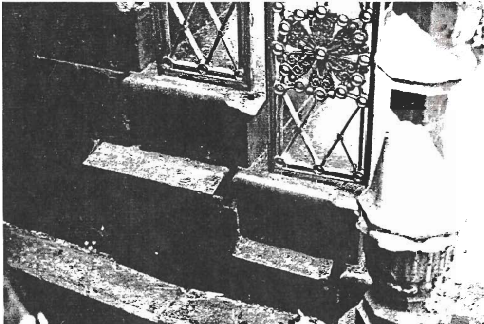
Figure 133 North Entrance Stone Stairs.
