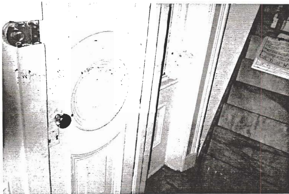
Figure 55 First Floor South Entry Door ("Star") Hardware.*
