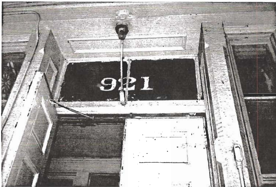
Figure 135 First Floor North Entrance Door Transom from Exterior.*
