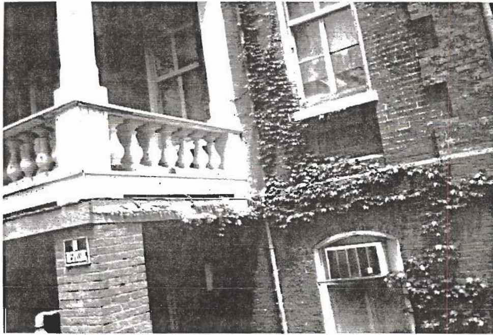
Figure 140 Side View of South Portico.*
