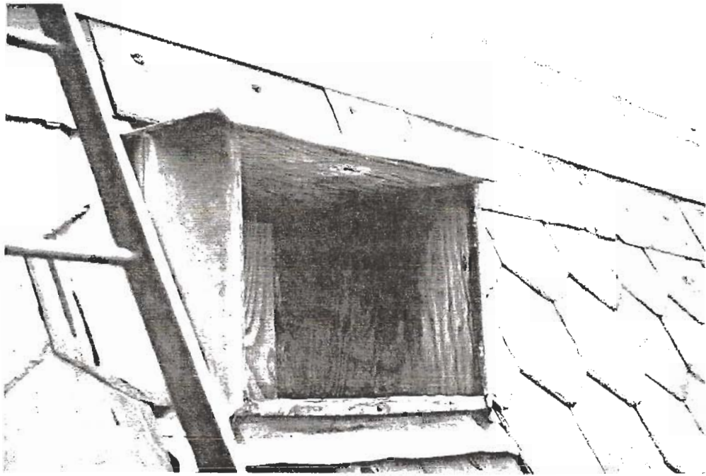
Figure 92 West Elevation at Mansard Roof Showing Typical A/C Opening.
