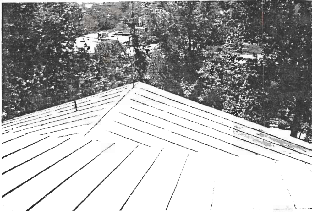
Figure 106 South Pediment Metal Standing Seam Roof.
