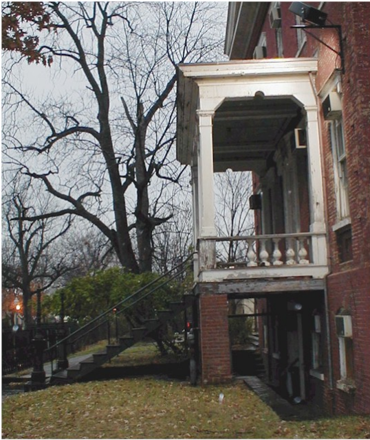
Main Exterior Staircase and Portico
