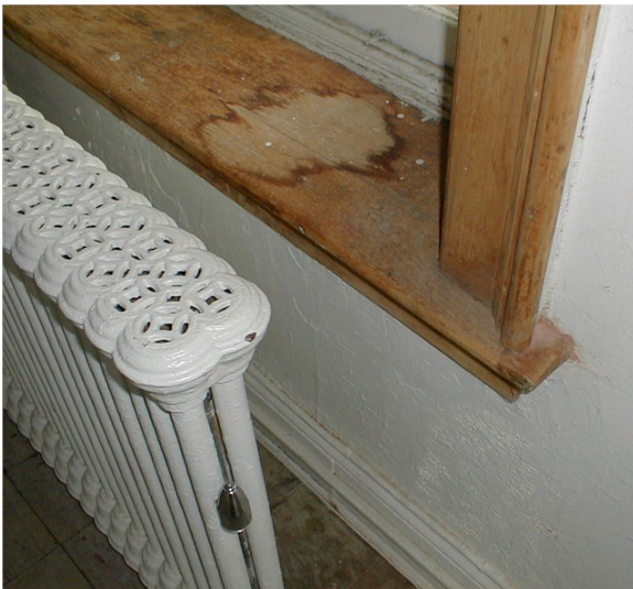
Radiator and Window Casing
