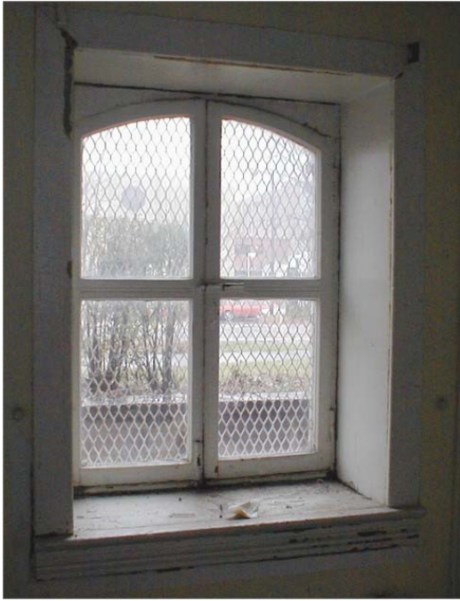
Basement Type 2 Windows
