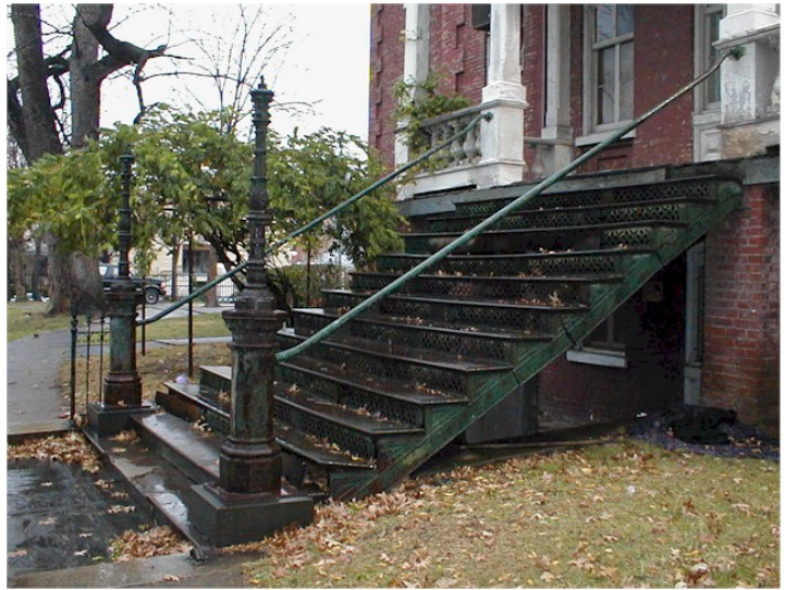
Main Exterior Staircase
