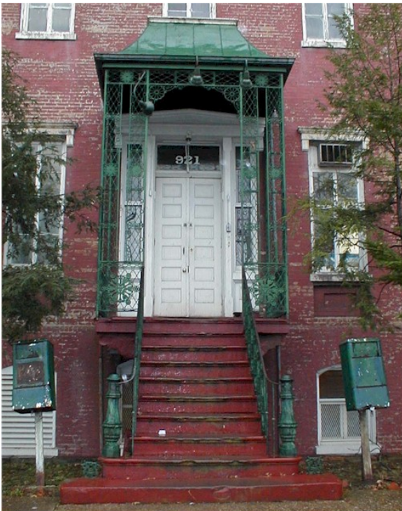
North Façade Staircase and Metalwork
